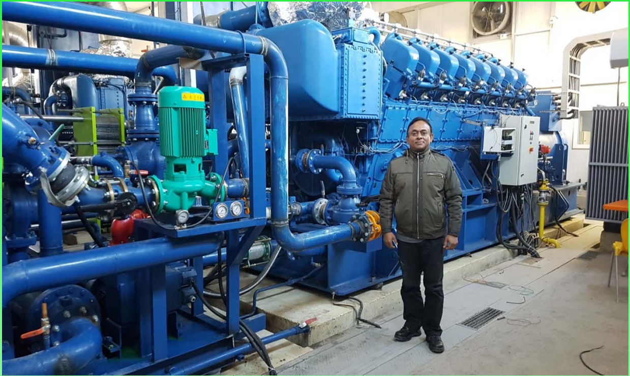
NATURAL GAS GENSET BEING MODIFIED FOR NOX COMPLIANCE
